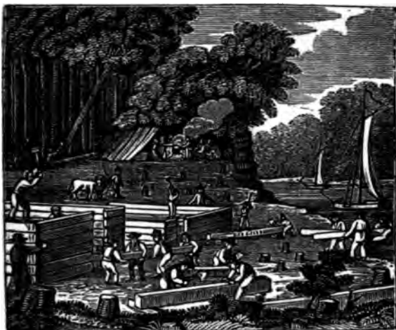
Building of Jamestown. P. 45.
